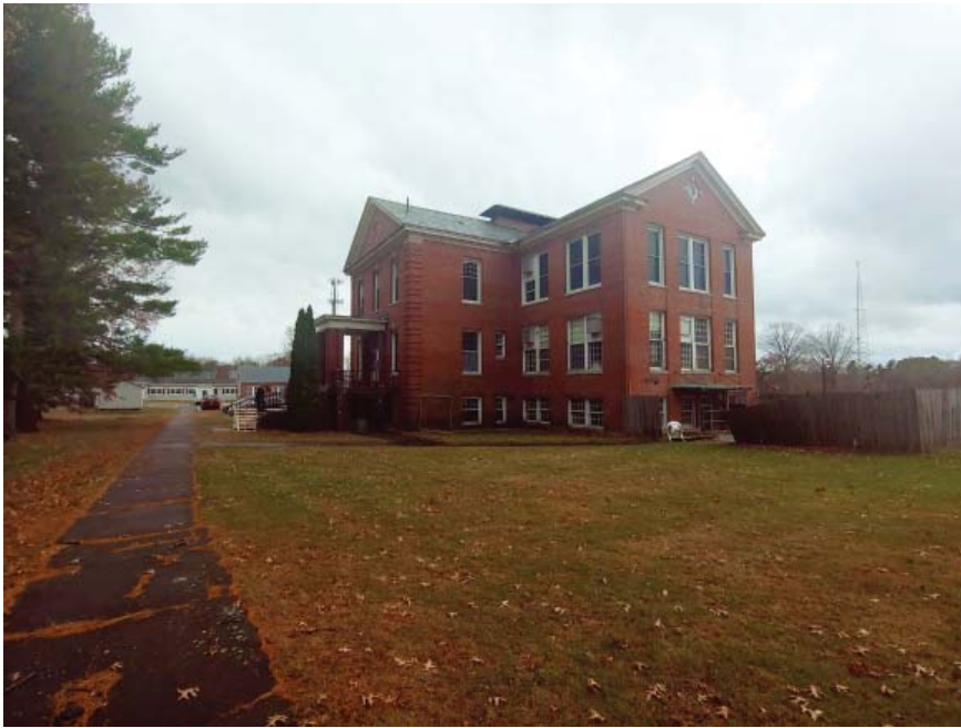
North-east of building from walkway.
