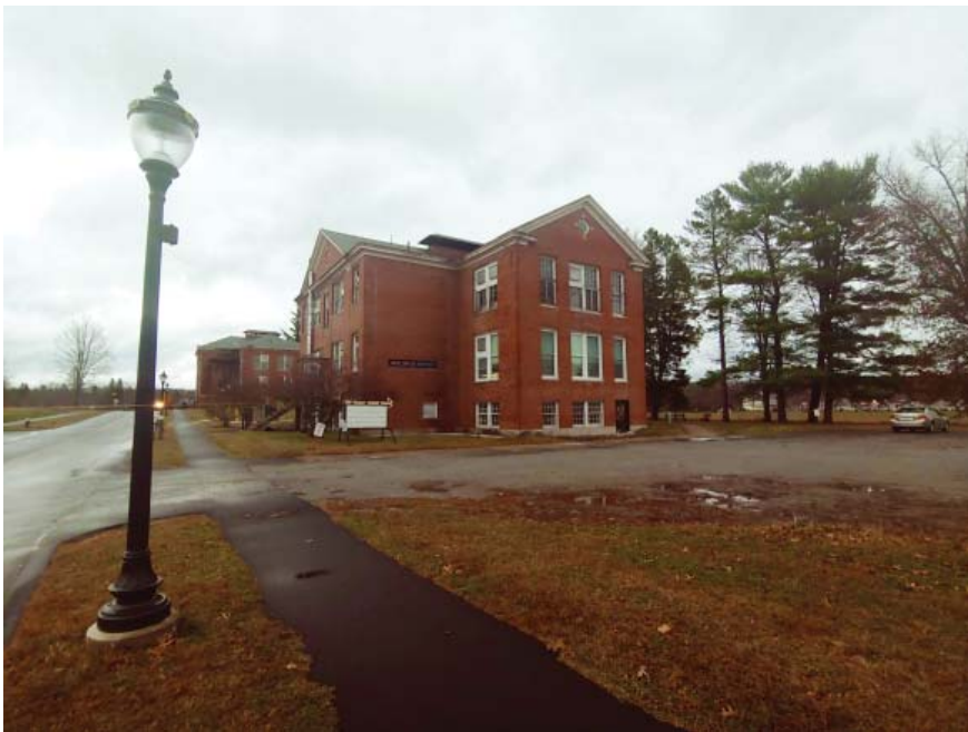
South-west of building from Berkshire Ave.
