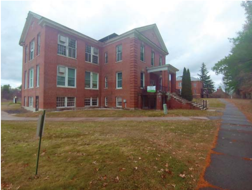
South-east of building from walkway.
