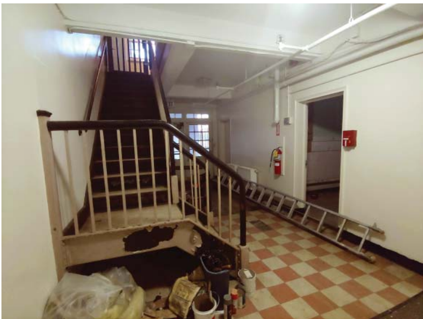
Main stairs on Ground Floor.
