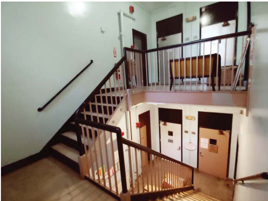
Main stairs between 2nd and 33rd floors.
