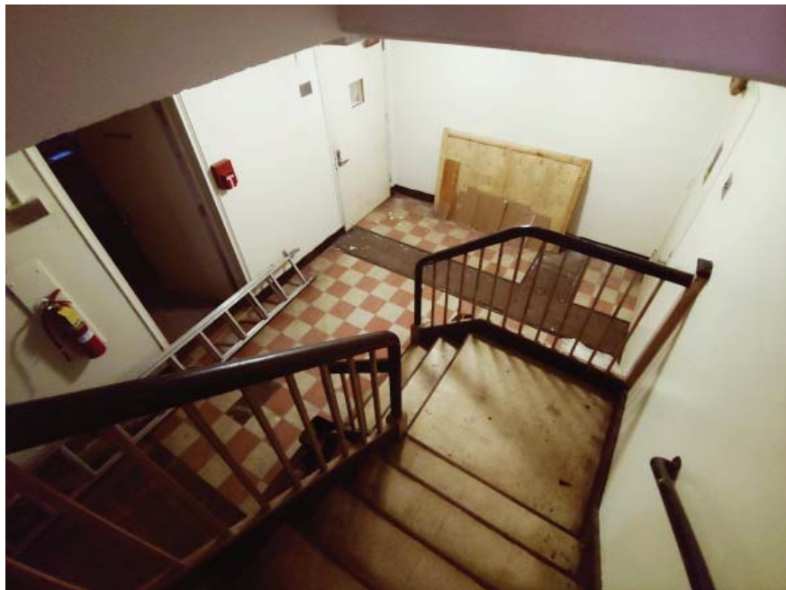
Main stairs looking down to Ground Floor.
